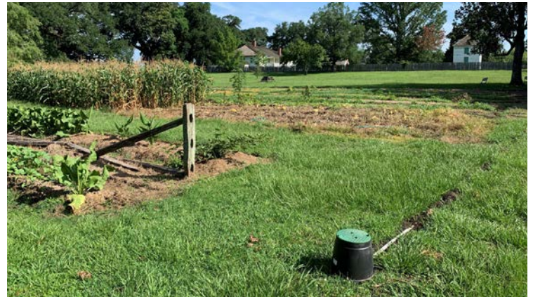
Camm Morton and Gee Gee Hargon recently installed an automatic watering system for the newly planted vegetable garden on the Magnolia Mound grounds. It was no easy feat! (Photo by Camm Morton)
